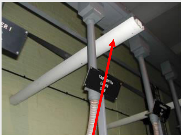
Above Circuit Breakers Cable Troughs (Cement)
