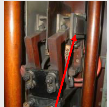
Circuit Breaker Main Isolator (Cement Flash Guards)
