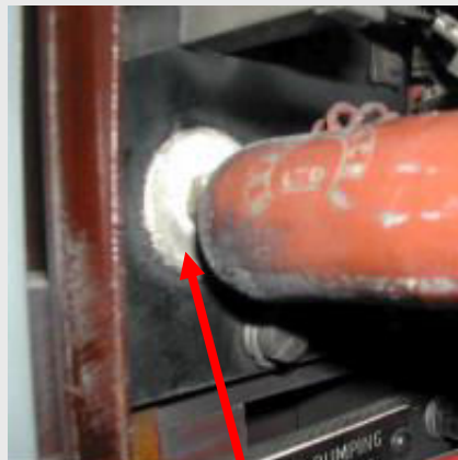
Circuit Breaker, Washer to Resistor
