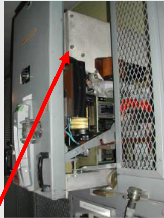
D.C. Circuit Breaker Arc Chute
